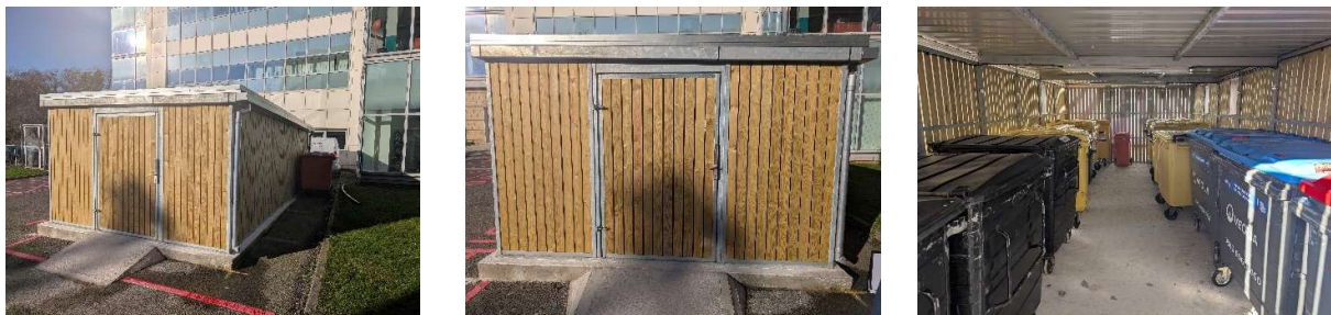
Figure 3 – Singleton Campus: External Euro 1100L bin covered compounds
