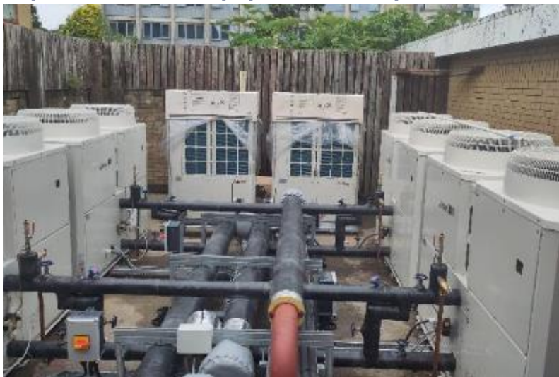
Haldane Building, air source heat pump
