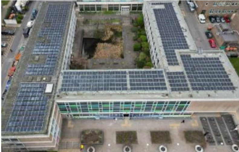
Glyndwr solar array, part of 1800 panel install
